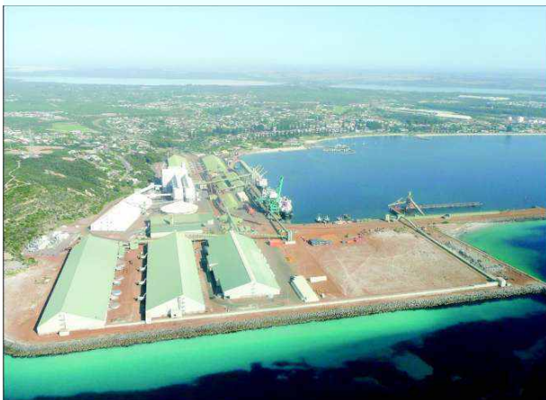
THE New Esperance Port expansion is expected to be located in the vicinity of Berth 3, the vacant area to the right of the photo, but will not affect ongoing operations of Cliffs' Natural Resource iron ore exports.
